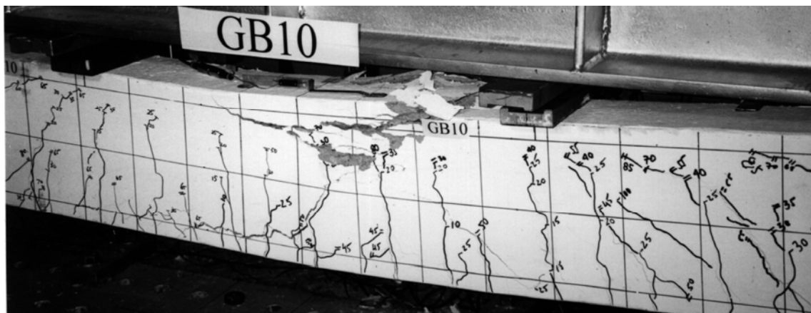
Plate 2 - Beam GB10 - Flexural failure at midspan
